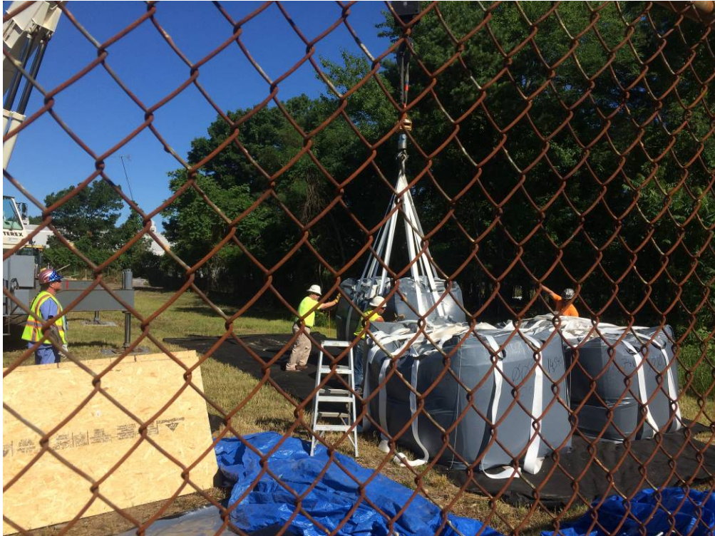
Photograph 5 – Excavated soil packaged in SPS Packaging Bags
