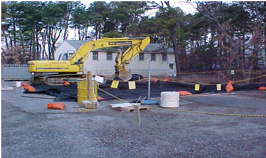
Picture 1: Concrete Pad Excavation Area Behind Building 650
