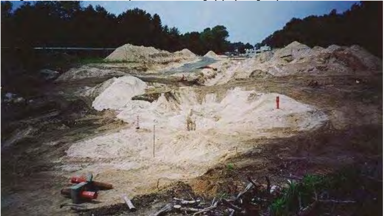
Picture 2: Outfall area on 6/27/02, showing additional excavations, and Building 650 in the background with the excavation path of the discharge pipe (facing SW).
