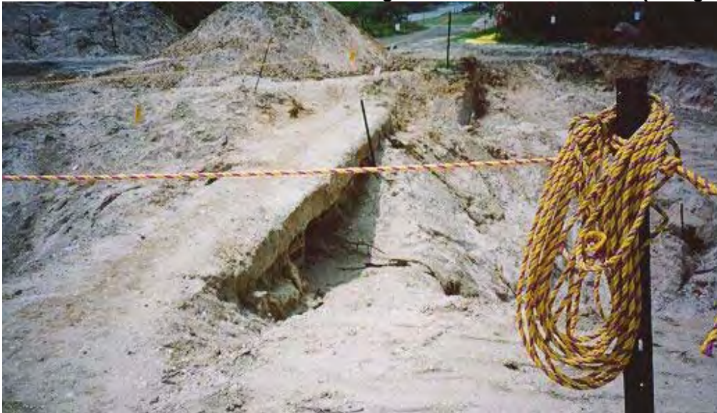
Picture 4: Electrical conduit with remaining subsurface contamination (facing S).
