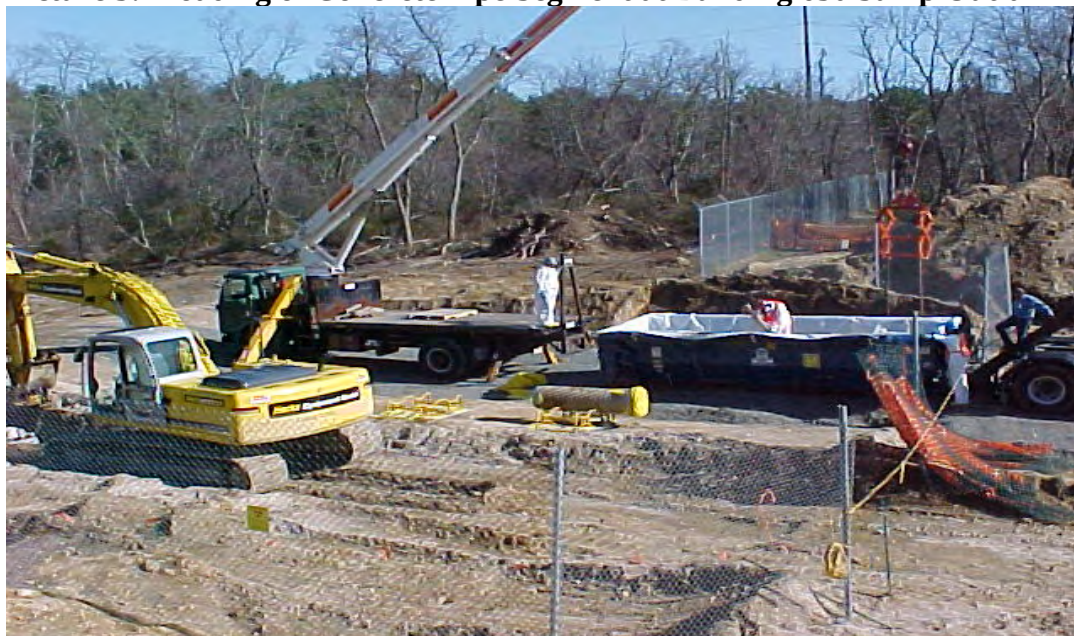
Picture 3: Loading of Concrete Pipe Segment at Building 650 Sump Outfall
