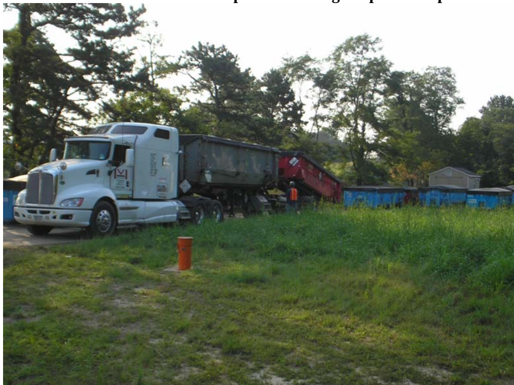
Photo 4: Rolloffs being loaded for transportation to disposal facility
