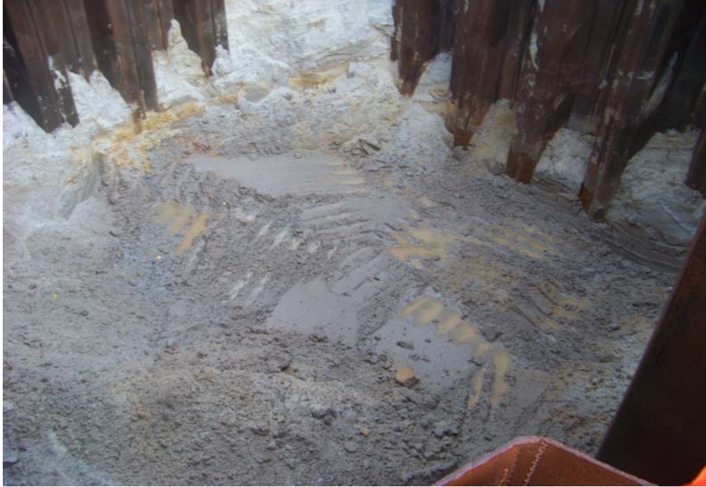
Photo 5: Bottom of Excavation upon completion of excavation
