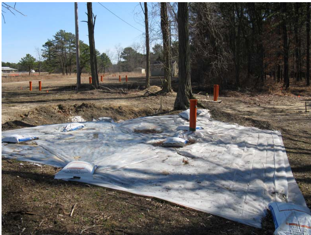
Photo 1: Approximate 25'x 25' Source Area Covered with Plastic prior to excavation (Well 085-353 in Center)
