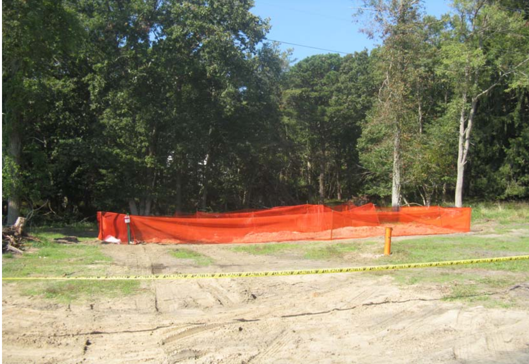
Photo 3: Excavation Completed awaiting endpoint samples
