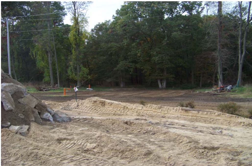
Photo 6: Area after Excavation was Completed and Backfilled
