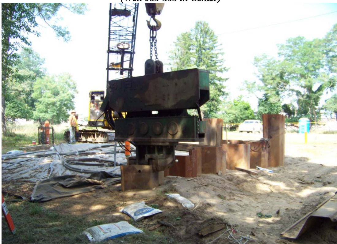
Photo 2: Shoring Installation
