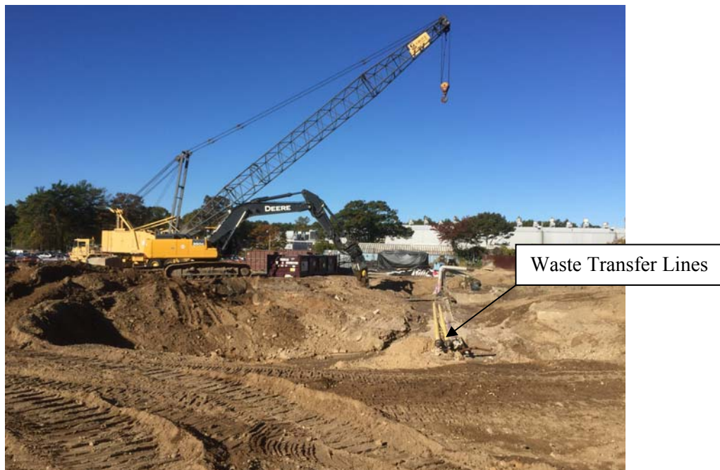
Photograph 7 – Waste Transfer Lines Removal
