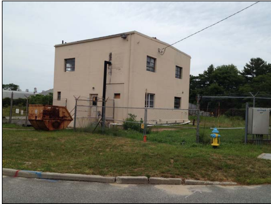
Photograph 1 – View of Building 811 Looking Northwest
