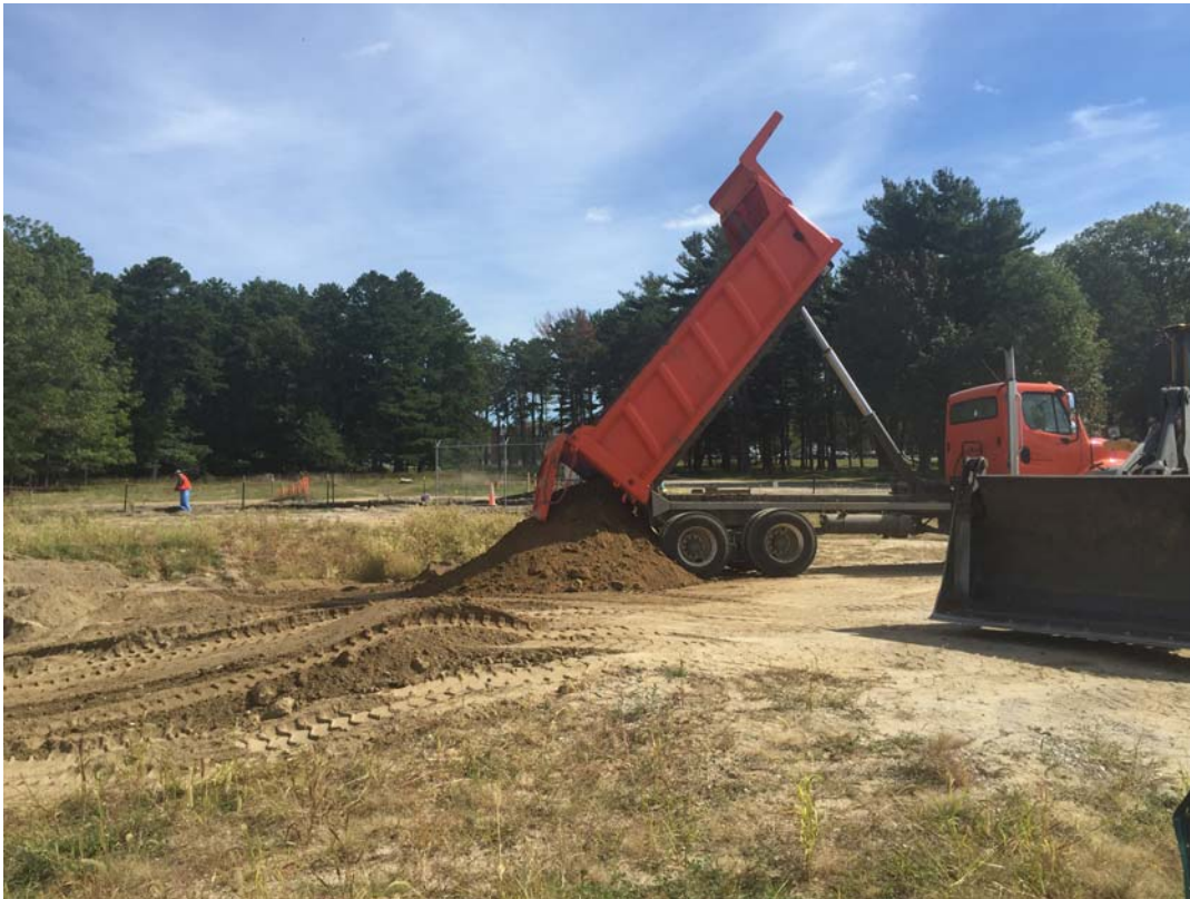
Photograph 11 – Placing clean fill at previous location of Building 811.
