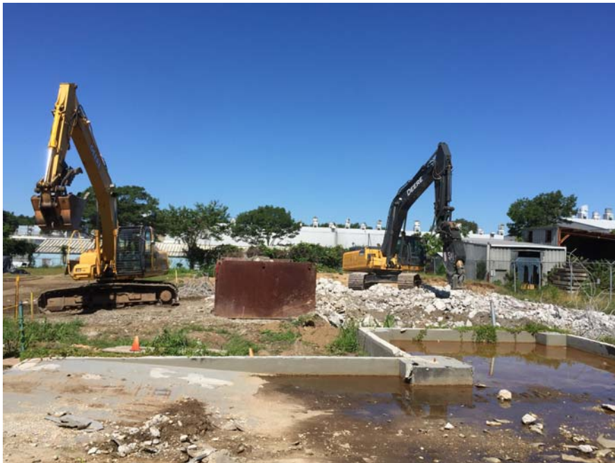
Photograph 6 – Demolition of AST Concrete Supports
