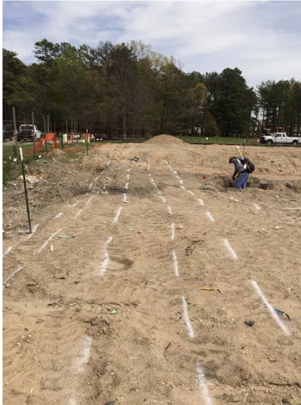
Photograph 9 – Performing Radiological Walkover Survey in SU-1
