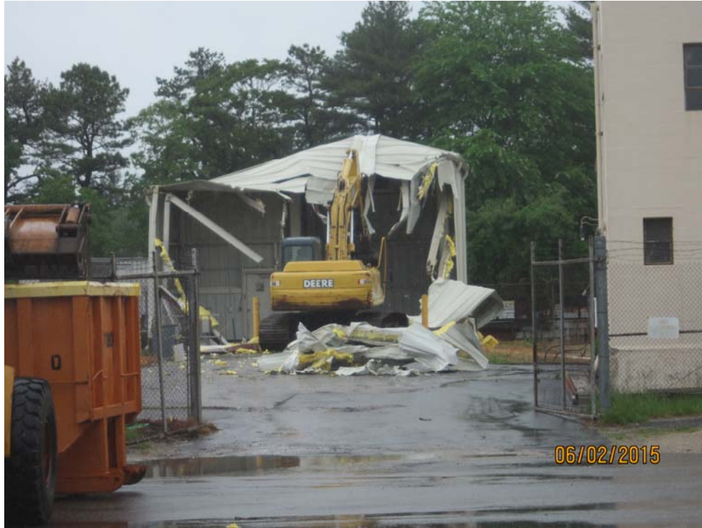
Photograph 3 – Demolition of Building 810
