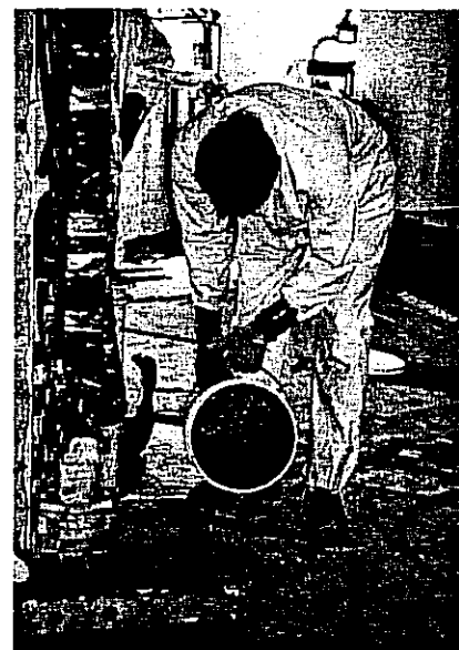
Figure 5-13. Backfilling with sand and CS.
