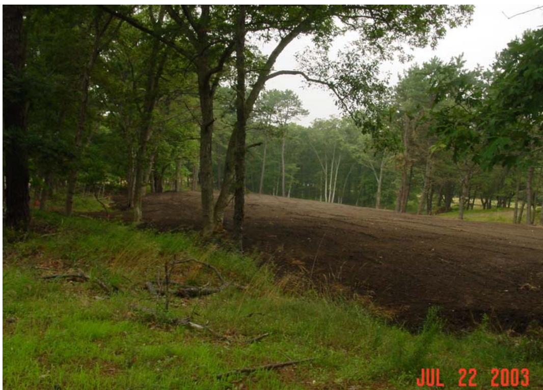
Photograph 5 – The Ash Pit area after the 12-inch topsoil cap has been installed
