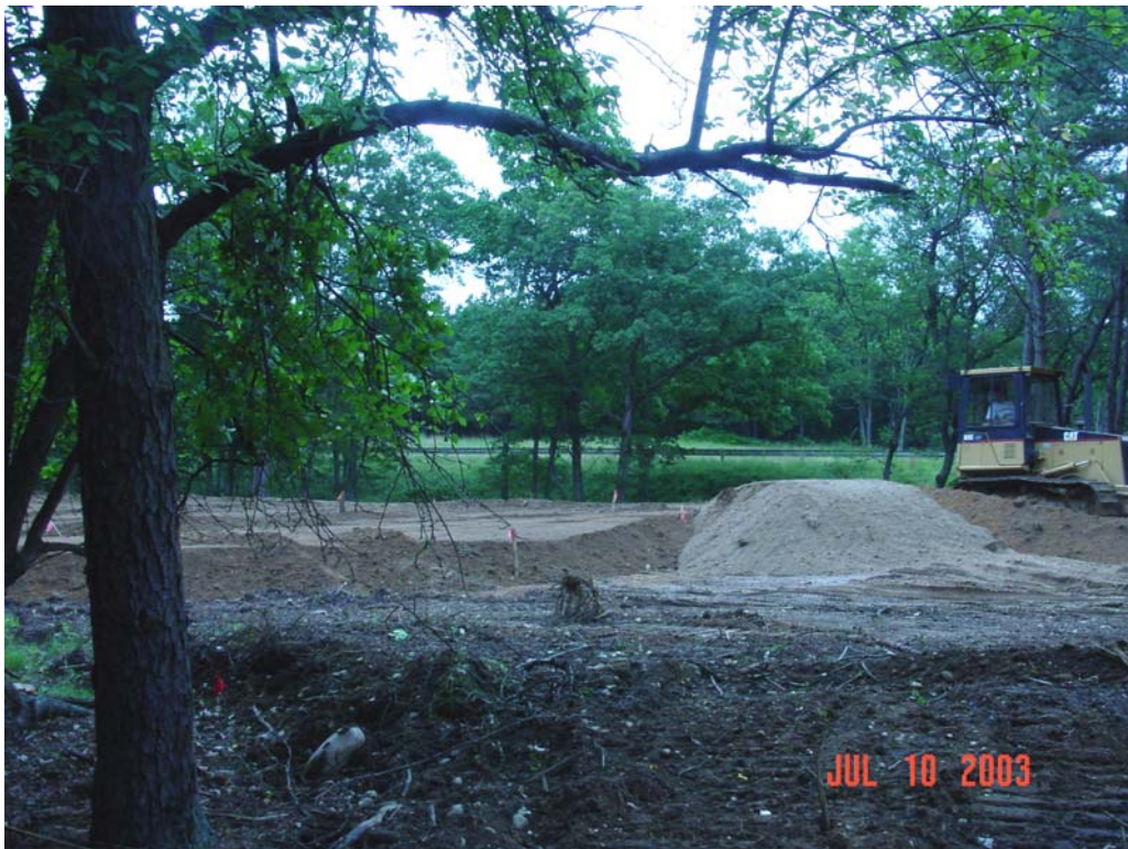
Photograph 4 – Clean fill being graded at the Ash Pit
