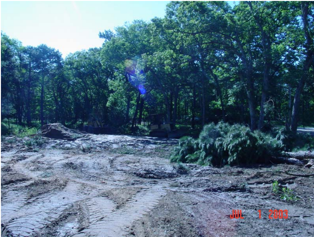
Photograph 1 – Clearing of trees and brush from the area requiring the soil cap.
