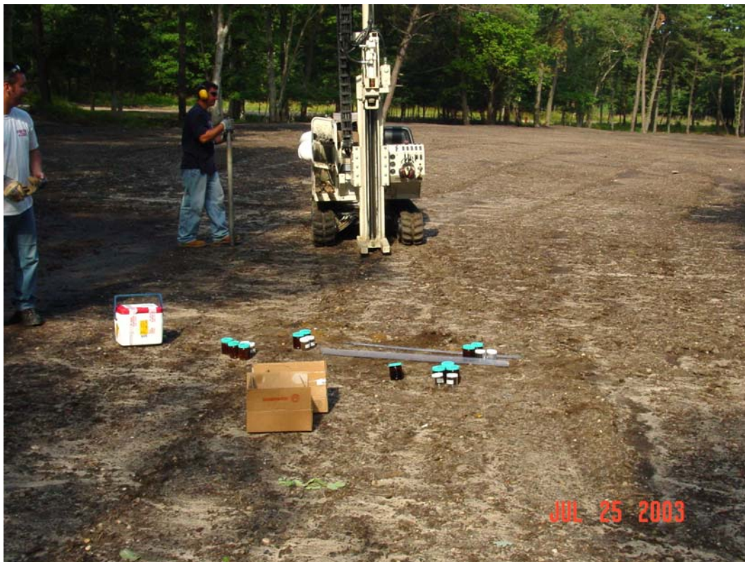
Photograph 6 – Verification sampling of cap depth and soil analysis
