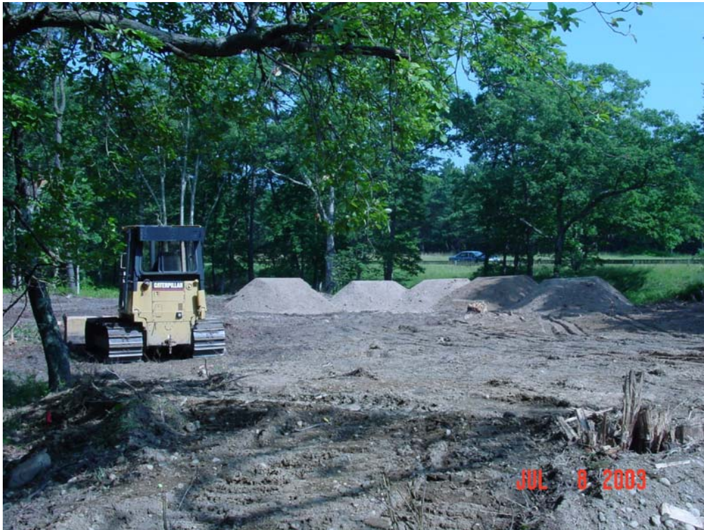
Photograph 3 – Clean fill staged prior to grading over the Ash Pit area
