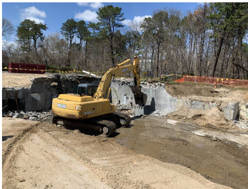
Photograph 7 – Removal of the Hot Laundry sump floor during Phase II.
