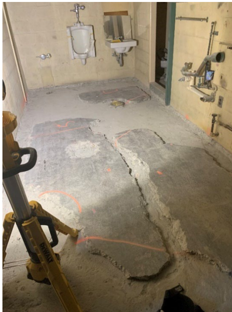
Photograph 2 – Portions of fixed radiological contamination removed from Hot Laundry side of Building 650.
