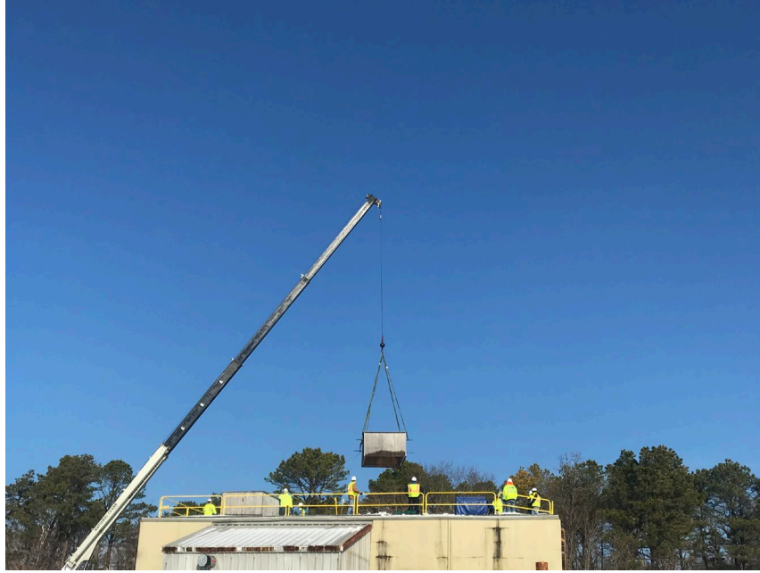
Photograph 3 – Removal of one of three T1-11 fan enclosures on the roof the Building 650 High Bay.
