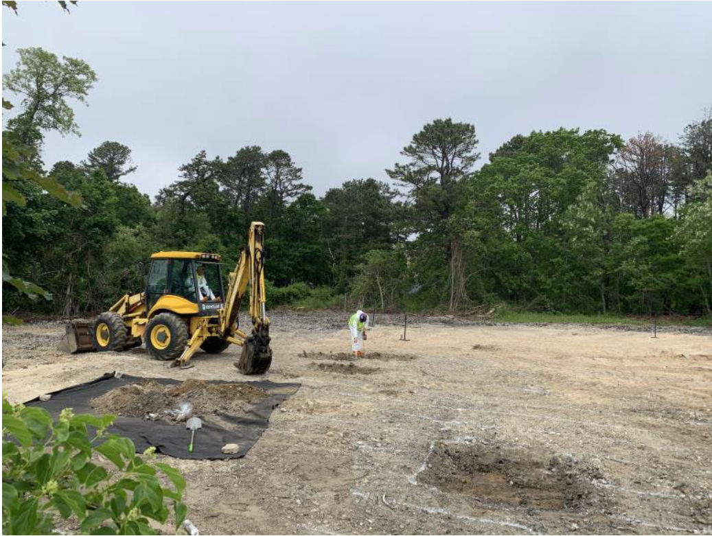
Photograph 8 – Backhoe excavating radiological hotspots and scanning areas with NaI detector.
