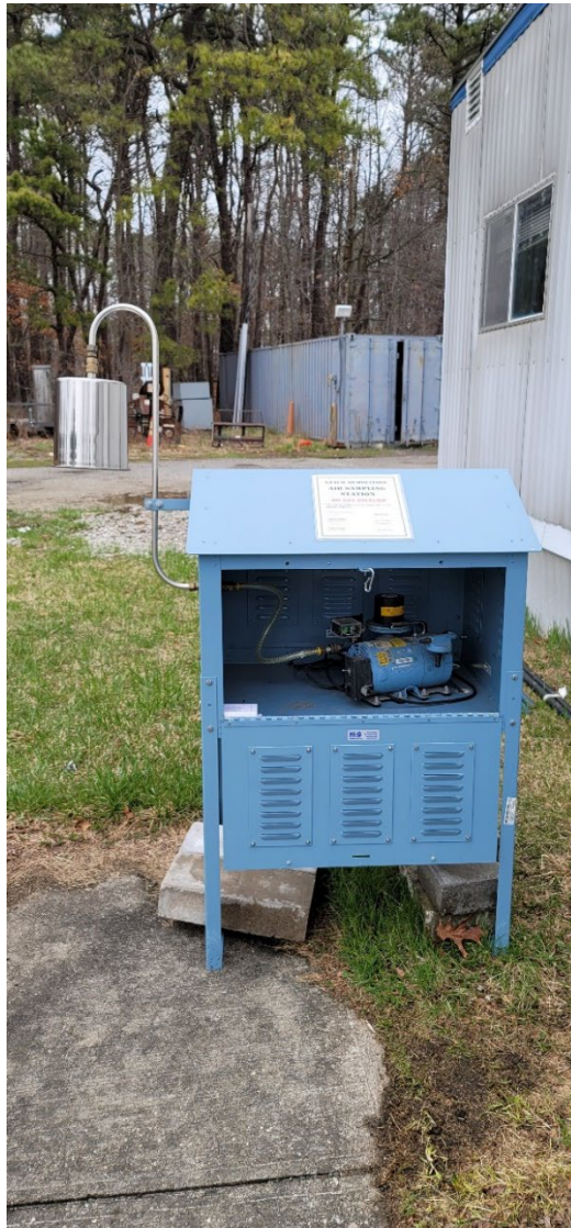
Photograph 13 – Air sampling station for radioactivity.
