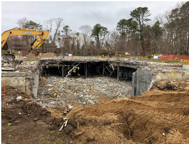
Photograph 6 – Demolition of the Hot Laundry 1 st floor during Phase II.
