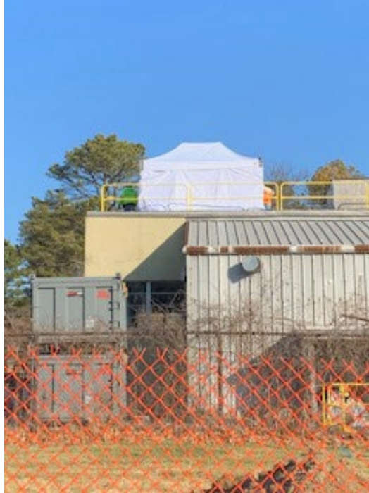
Photograph 4 – Containment tent constructed for asbestos abatement at southwestern T1-11 fan enclosure.
