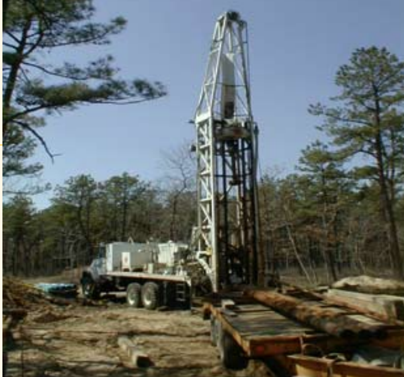
One of the drill rigs used to install the off-site groundwater sampling and treatment wells.
