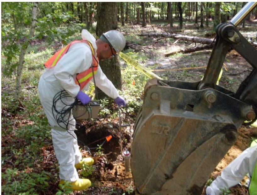
Photograph 2 – Remediation of discrete area of elevated radiological activity within the LISF area.
