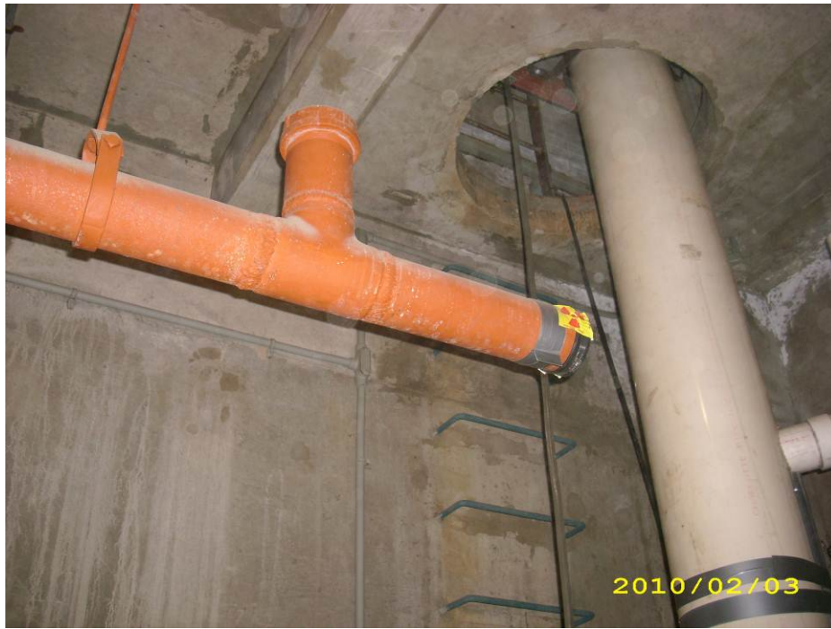
Photograph 2 – Temporary Stack Drain Sump and Old Stack Drain Line in the Basement of Building 704
