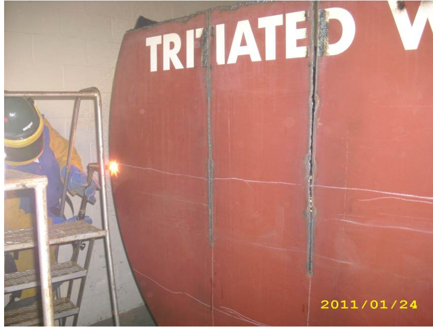
Photograph 5 – Cutting 5,000-gallon tritiated waste tank with torch
