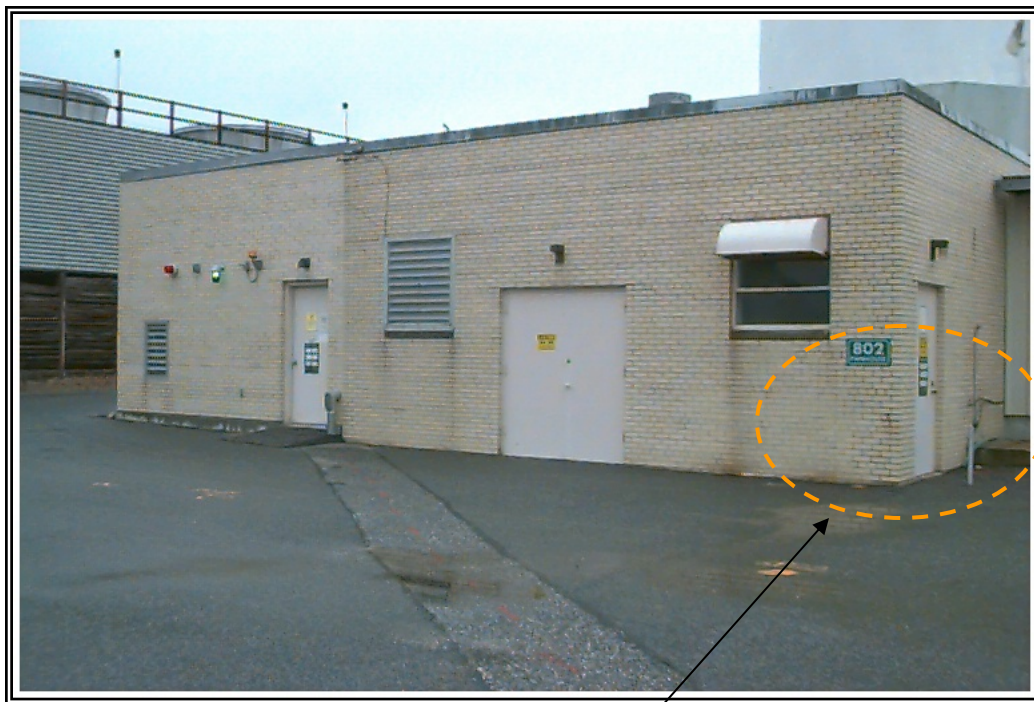
Picture of Building 802 prior to D&D Approximate location of spill site
