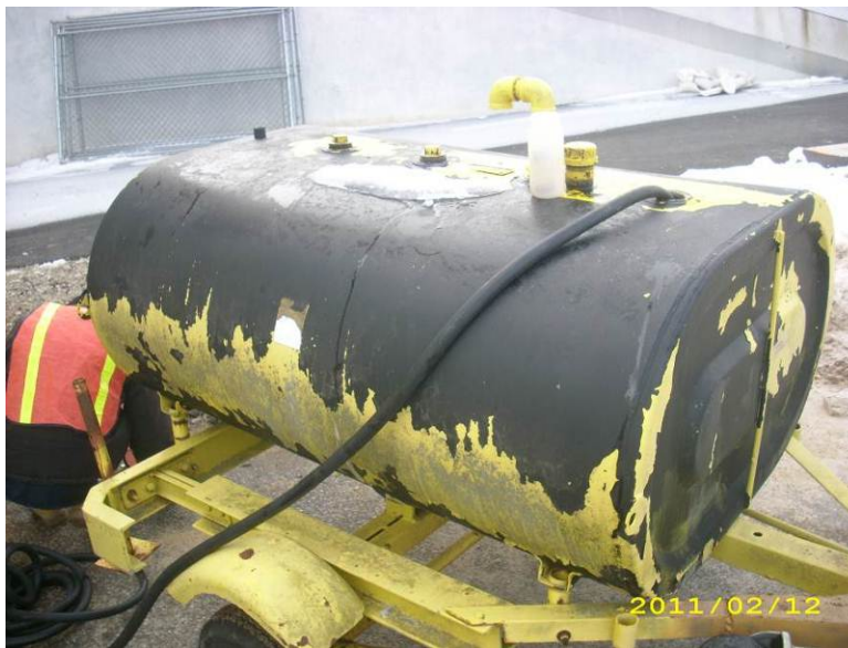
Photograph 6 – Cleaning out and removing 275-gallon diesel fuel tank
