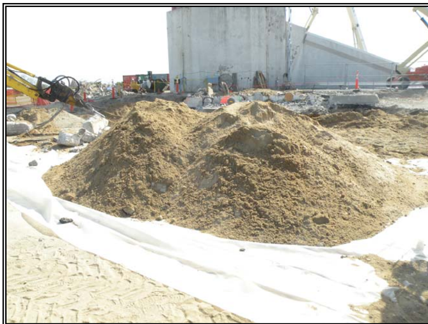
Approx. 3 cubic yards of contaminated soil removed.
