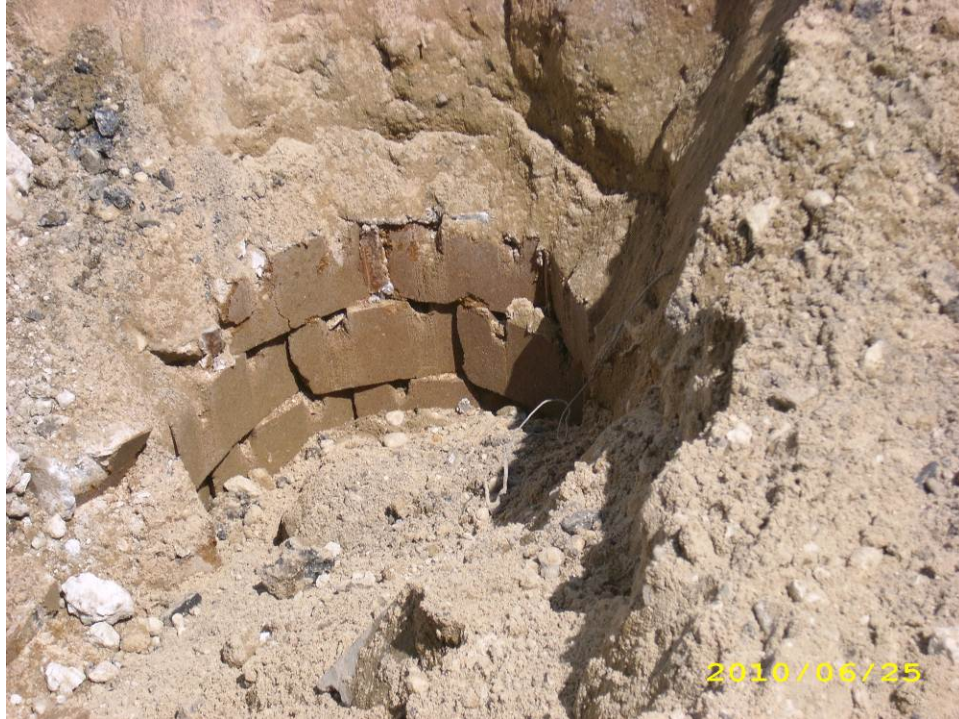
Photograph 10 – Drywell discovered adjacent to southeast corner of Building 704
