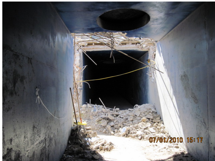
Photograph 9 – Interior of underground plenum
