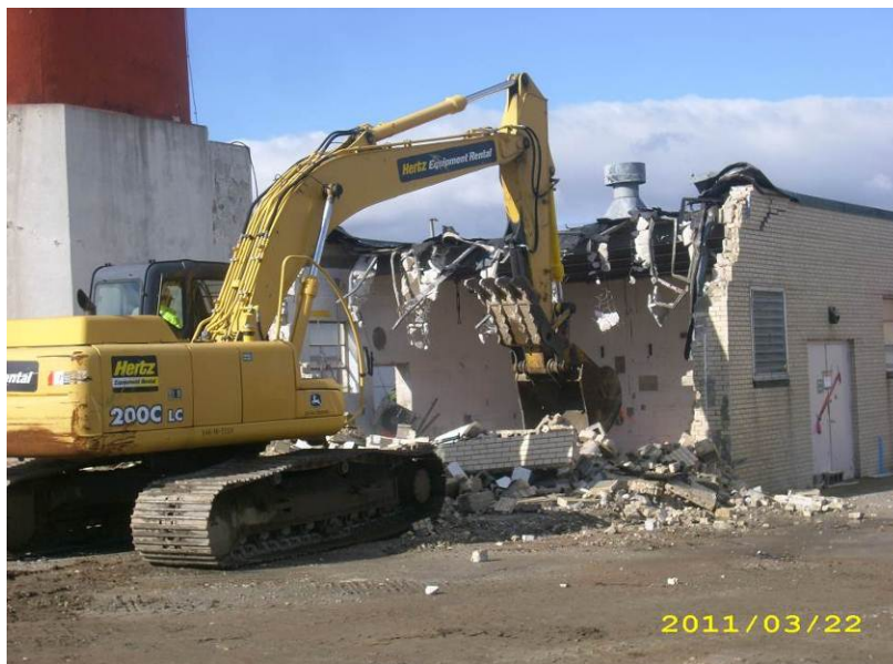
Photograph 7 – Demolition of Building 802
