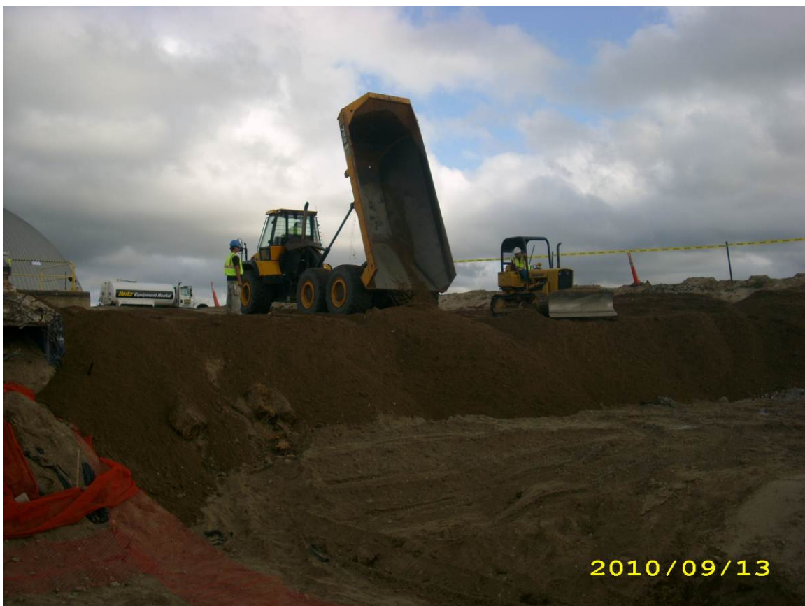
Photograph 13 – Placing clean fill at previous location of Building 704.
