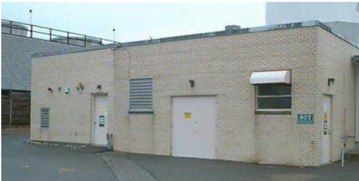
Photograph 3 – View of Building 802
