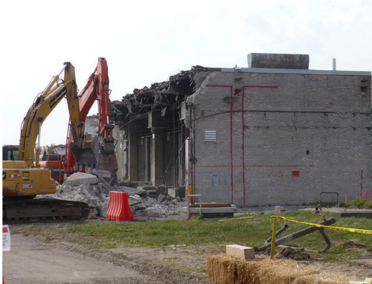
Photograph 4 – Demolition of the southern half of Building 704
