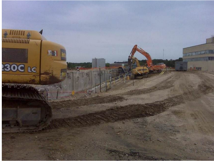
Photograph 8 – Demolition of the Building 704 underground plenum
