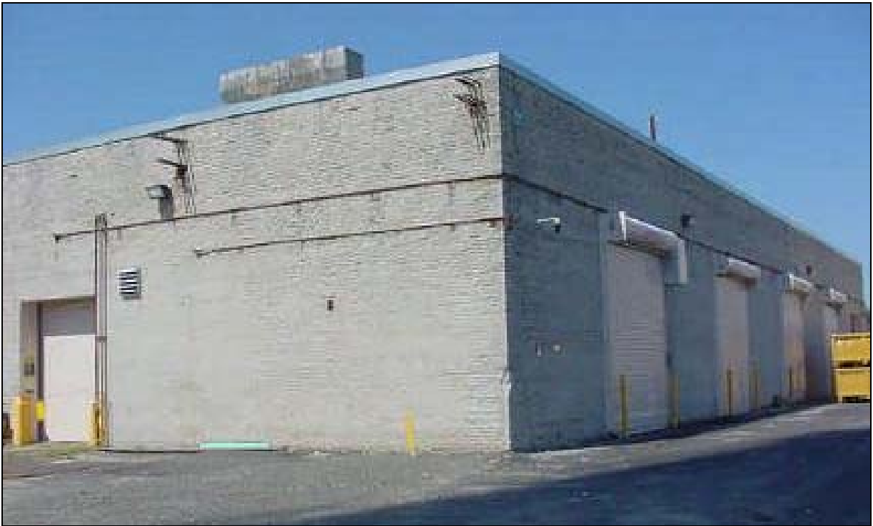
Photograph 1 – View of Building 704 Looking West
