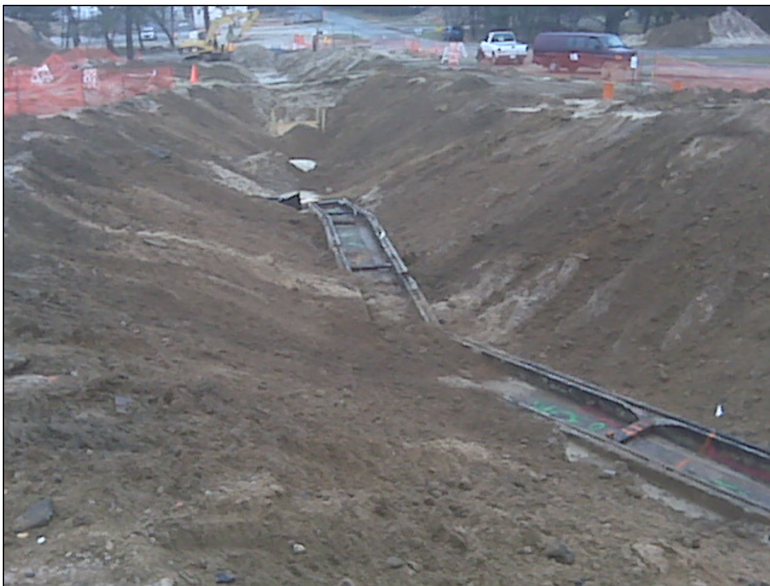
Photograph 4 – Segment of Phase 1 concrete culvert left in ground
