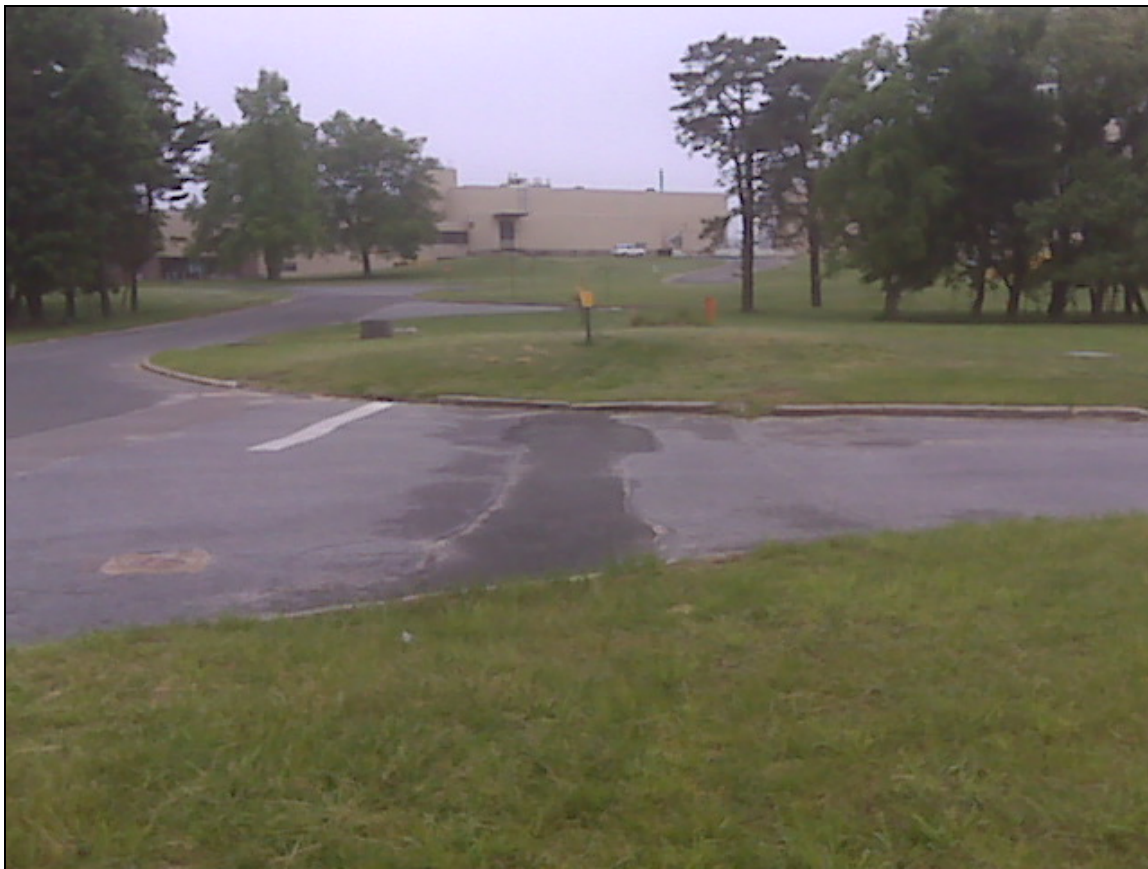
Photograph 1 – Pre-excavation conditions at the Waste Transfer Lines site (Phases 1-3)
