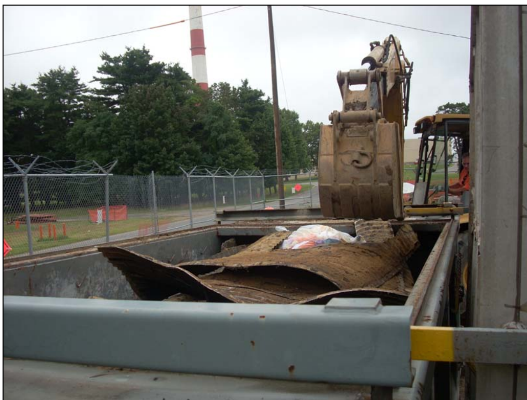
Photograph 5 – Packaging of Waste Transfer Lines debris.
