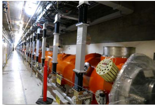
10 of 35 CMs installed in SLAC tunnel
