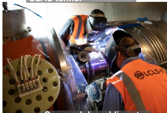
Cryomodule welding at SLAC
