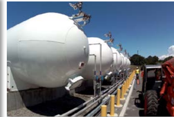
Cryopant tank farm at SLAC
