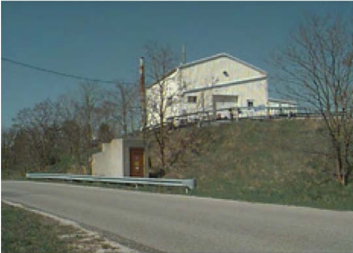
Figure 2. The BLIP facility.
