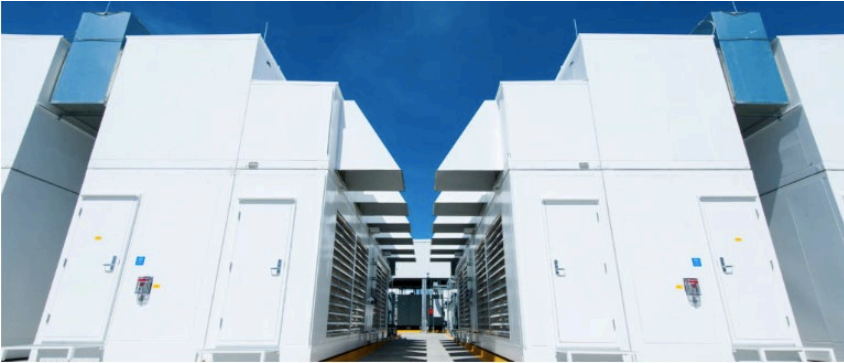
Microsoft Datacenter, Quincy
