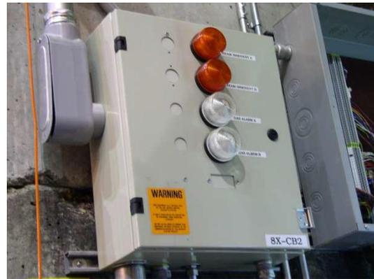
Beam Imminent Signal: Orange Strobe Light and an Audible Alarm
