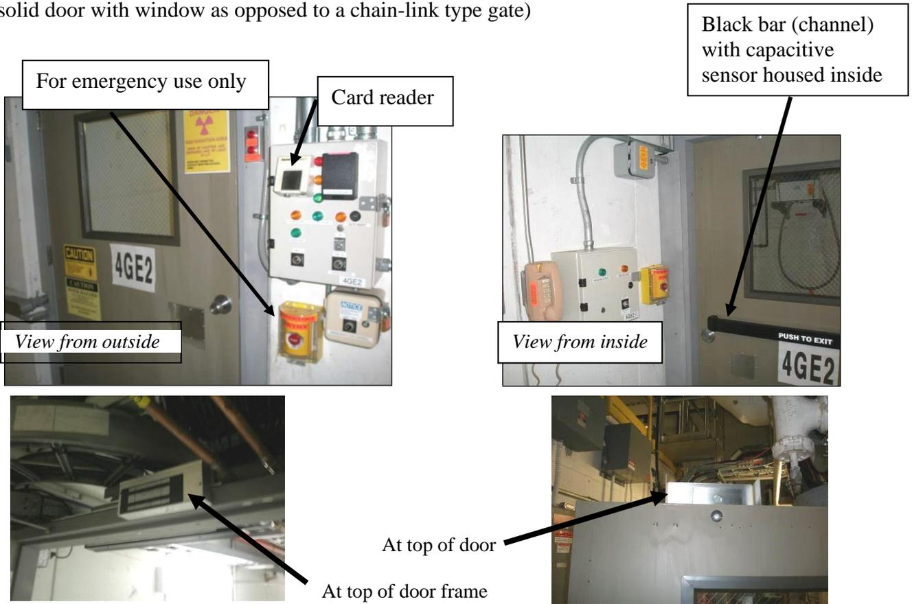
With this newer type door, there is no mechanical door latch mechanism so you do not turn the door knob to enter or exit. The door is held closed by a magnet installed at the top of the door frame. To enter during Restricted Access Mode, place your RHIC card-key on the card reader (same as with the older type door). This releases the magnet and allows you to pull open the door.
