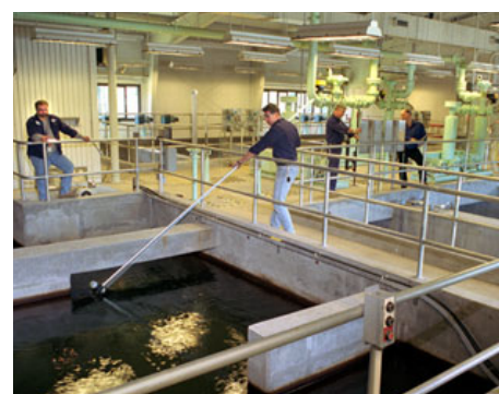
6. RETENTION TANK holds the water long enough to allow the chemicals time to react and form floc. To aid in the formation of floc, the water is then sent to a slow-mix tank. At the retention tank are: (from left) Steve Barcelo, Jack Kulesa (who is checking for floc particles), and Richard Lutz, plus Frank Masia.
