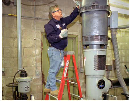
1A. WELLS 4, 6, and 7 provide source water high in iron that must be "finished" at BNL's Water Treatment Facility (WTF). At one of these wells, Phil Pizzo performs preventive maintenance on pump motor.
