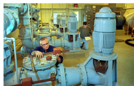
8. WET WELL stores the filtered water before it is pumped into the air-stripping towers. While Jack Kulesa (background) inspects the wet-well pump seals, Richard Lutz works on a check valve.
