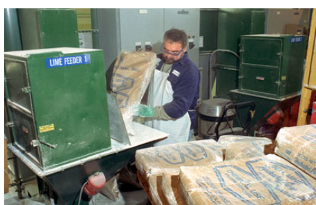
4. LIME is added after aeration (no. 3) and before retention (no. 6) to raise the pH and soften the water. Feeding lime into the hopper is Steve Barcelo.
