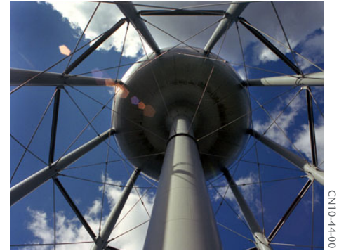
12. ONE-MILLION-GALLON WATER STORAGE TOWER , as viewed from its base, is the larger of the Lab's two water towers. Built in 1985, and located at Cornell and North Sixth Street, this tank is 126 feet above the ground; its bowl is 75.5 feet in diameter. Located next to Police Headquarters, Bldg. 50, the other water storage tank holds 300,000 gallons and was built for the U.S. Army in 1941, when the site was Camp Upton. At a pressure of 55 to 70 pounds per square inch, water from the two towers is delivered on site via 45 miles of distribution pipe, which is a mix of cast iron dating from World War II Camp Upton, transite, plastic, and cement-lined ductile iron. When distribution pipe is added or replaced, cement-line ductile iron is used.
