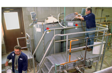
5. POLYMER is also added to the water after aeration to aid in a process called flocculation, whereby very small hydroxide particles stick together to form larger particles, called floc, which are more easily settled and removed (see no. 6). The polymer is mixed with the water in a rapid-mix tank. Steve Barcelo (left) is seen measuring the polymer, while Tom Boucher prepares to mix.
