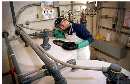
2. CHLORINATION of water from wells 4,6, and 7 is performed at this point using sodium hypochlorite to kill bacteria and oxidize the iron in the water. Iron removal by oxidation and filtration reduces the water's iron concentration from 3 to 4 milligrams per liter (mg/l) to the "finished" water's 0.03 mg/l. Inspecting a liquid sodium hypochlorite storage tank is Joe Tullo.
