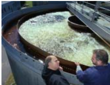
3. AERATION TANK reduces carbon dioxide gas and aids in the oxidation of iron. At the aeration tank, Steve Barcelo (right) describes the action to Frank Masia.
