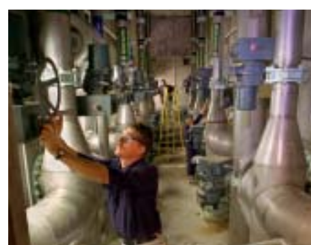
7. FILTRATION is performed, using what is called a rapid sand filter made up of eight filter cells containing sand and anthracite. Inspecting the valves in the filtration valve gallery are: (front to back) Jack Kulesa, Richard Lutz, and Steve Barcelo.
