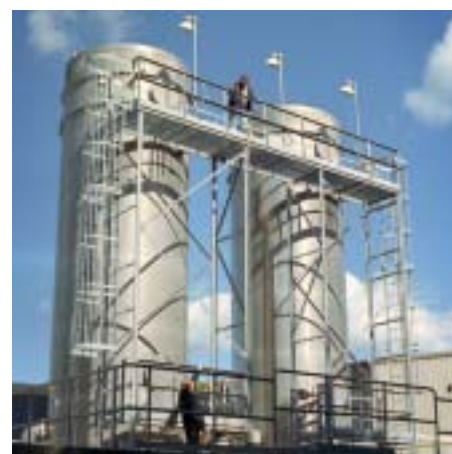
9. AIR-STRIPPING TOWERS remove any volatile organic compounds (VOCs) from the water undergoing the WTF process by spraying the water down over whiffle ball-like fill while air flows upward through the water spray. Inspecting the towers from the top is Steve Barcelo. Frank Masia looks on from below.
