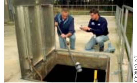
10. CLEAR WELL stores up to 250,000 gallons of what is now called "finished" water before its final chlorination and distribution. Seen taking a water sample at the clear well are Jack Kulesa (left) and Richard Lutz.
