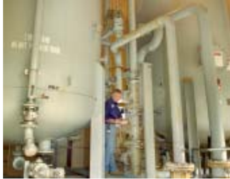
1B. CARBON FILTRATION AT WELLS 10, 11, and 12 is designed to remove volatile organic compounds before the low-iron water from these three wells directly enters the drinking-water distribution system. Noting the pressure of the carbon filtration system is Richard Lutz.
