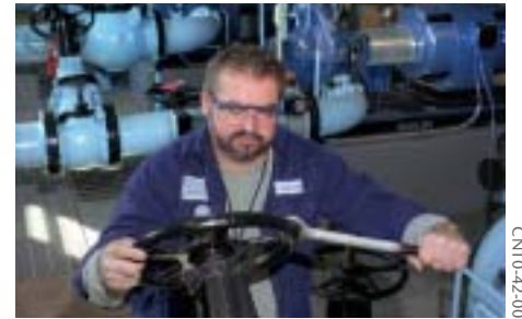
11. HIGH-SERVICE PUMPS send finished water from the WTF to the two water towers on site. Adjusting the flow rate of a high-service pump is Steve Barcelo.
