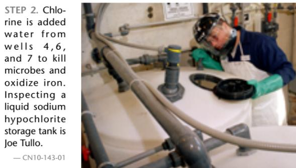
**STEP 2.** Chlorine is added from wells 4, 6, and 7 to kill microbes and oxidize iron. Inspecting a liquid sodium hypochlorite storage tank is Joe Tullo. — CN10-143-01
