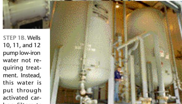
**STEP 1B.** Wells 10, 11, and 12 pump low-iron water not requiring treatment. Instead, this water is put through activated carbon filters to remove volatile organic compounds. It is then chlorinated and pH adjusted before entering the water distribution system. Noting the pressure of the carbon filtration system is Richard Lutz. — CN10-147-00
