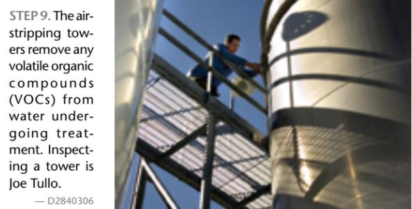
**STEP 9.** The air-stripping towers remove any volatile organic compounds (VOCs) from water undergoing treatment. Inspecting a tower is Joe Tullo. — D2840306
