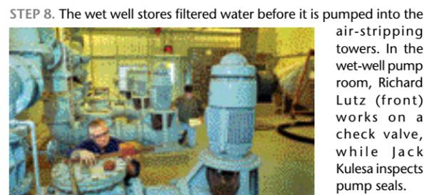
**STEP 8.** The wet well stores filtered water before it is pumped into the air-stripping towers. In the wet-well pump room, Richard Lutz (front) works on a check valve, while Jack Kulesa inspects pump seals. — CN10-38-00
