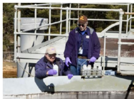
**STEP 3.** Aeration reduces carbon dioxide gas and aids in iron oxidation. At the aeration tank, Phil Pizzo and Greg Stawski sample the water. — D2850306
