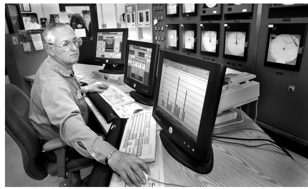
In the control room of BNL's Water Treatment Facility (WTF), Bldg. 624 on Upton Road, is Richard Lutz. — D2820306
