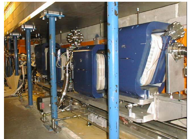
ATF bunch compressor installed in tunnel.
