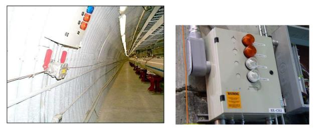
Beam Imminent Signal: Orange Strobe Light and an Audible Alarm
