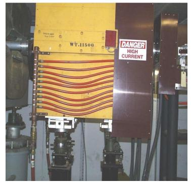
Orange tubing typical for magnet cooling water:
