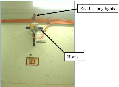
Beam Imminent Signal: Red Flashing Lights and an Audible Alarm
